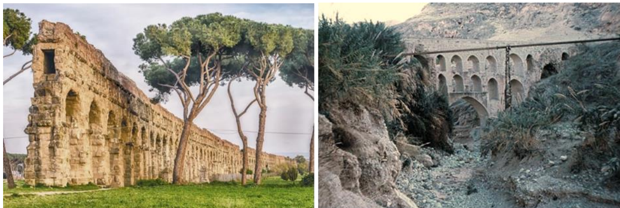
Figure 1. Parco degli acquedotti, Rome/Italy (URL1) – Roman aqueduct near Jericho (URL2)
