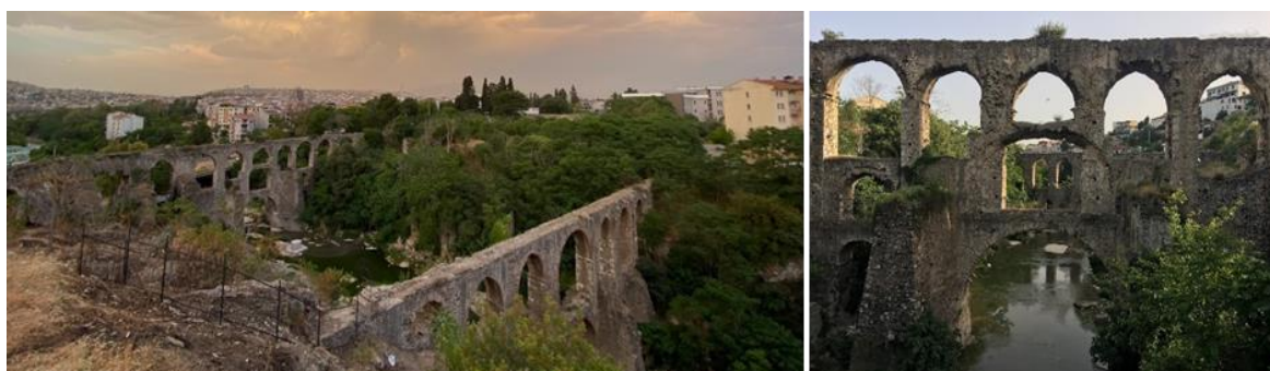
Figure 6. Kızılçullu Aqueducts covered in the study (Google Earth)
