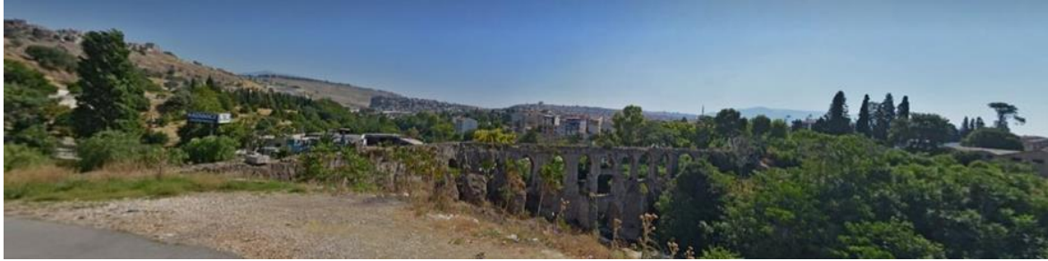
Figure 8. Panoramic photo of Kızılcıllu Aqueducts
